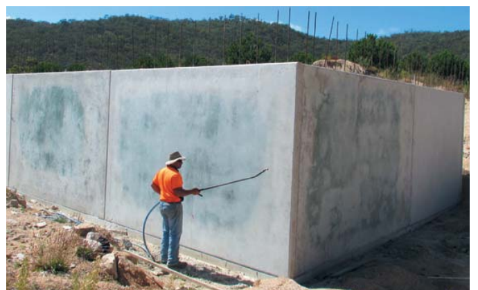
About to spray the underground wine cellar with bitumen
